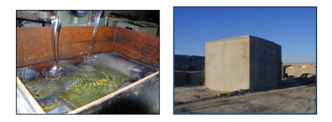
Figure 3-1. Macroencapsulation of Hazardous Debris
