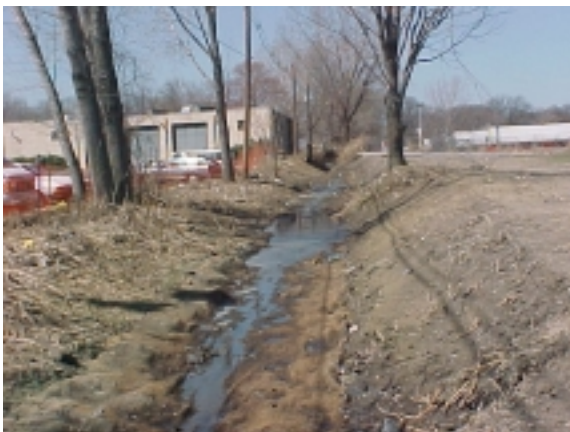
March 24, 2000 – View of Swale looking West after restoration activities.
