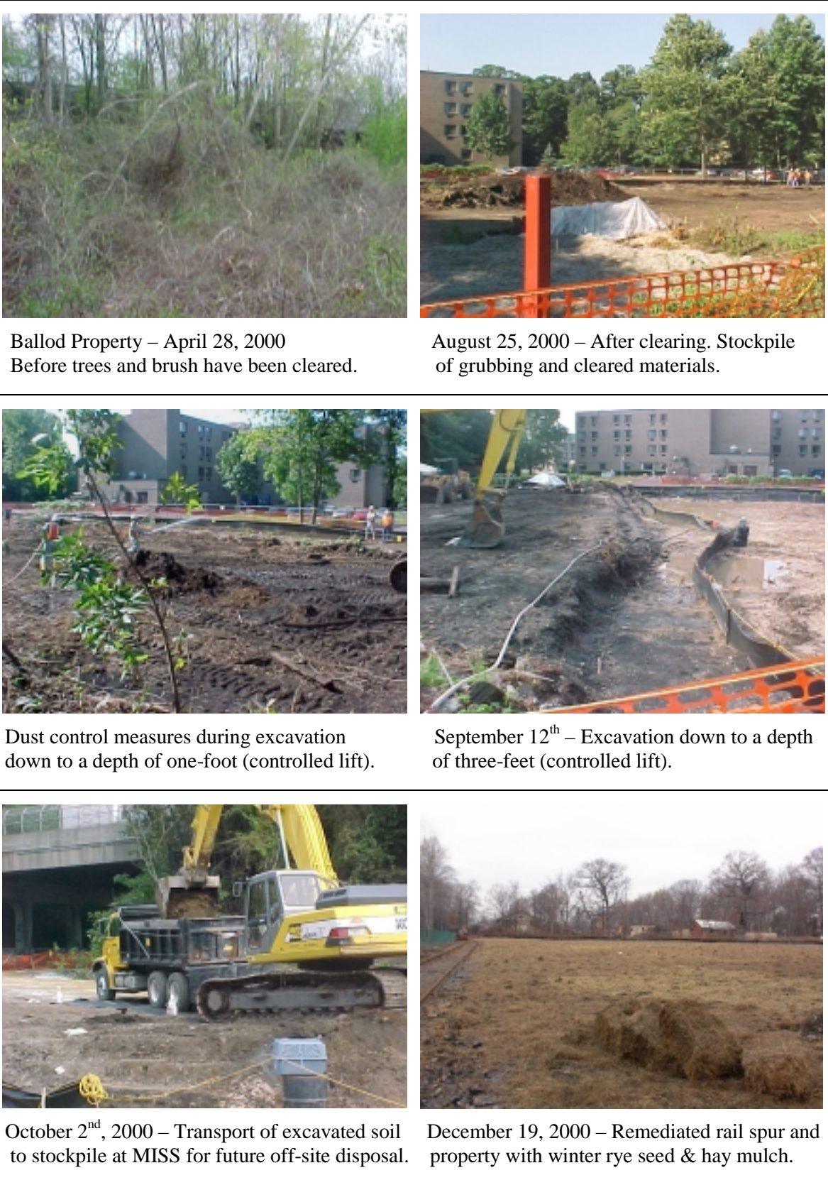
Figure 5 Ballod Property Remediation and Restoration – Selected Photographs
