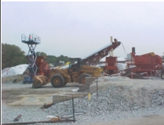
Gravel separated from acquisition soil. Material transported to soil staging area.
