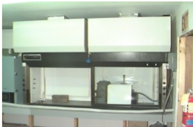
Grinding of soil samples is performed under the fume hood which exhausts to the HEPA filter.
