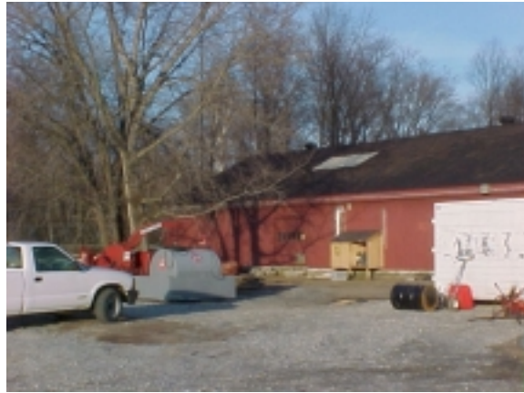
Building 76 on MISS – Location of Soil Sample Preparation Laboratory.
