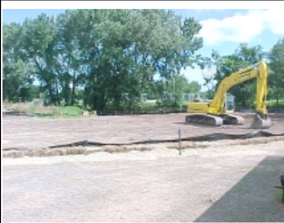
Soil acquisition area. First controlled cut. Kobelco excavator.
