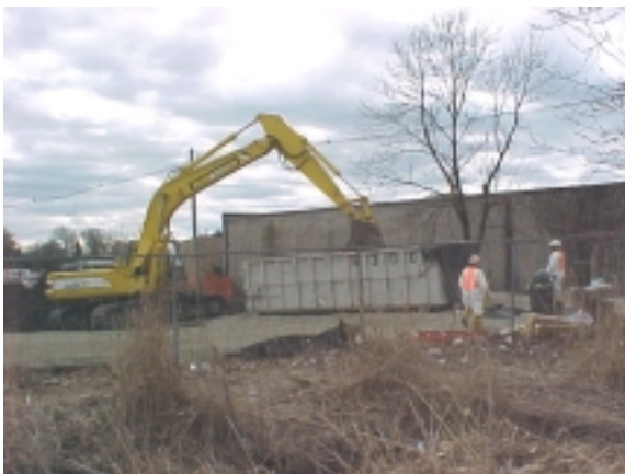
Excavated soils were placed into roll-off containers for transport to MISSS
