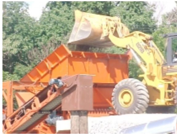
Acquisition soils fed into first hopper – Gravel Separation System (GSS)
