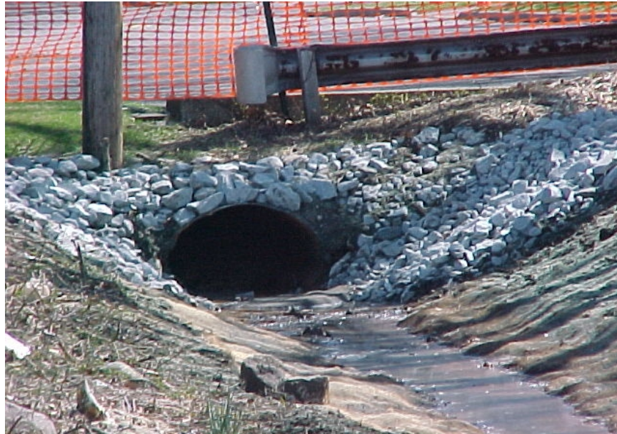
Photo C-1 View of the culvert at the terminus of West Howcroft Road.
