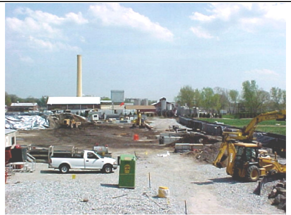
April 2001 – Westward view of MISS. Front-end loader removing soil from stockpile.
