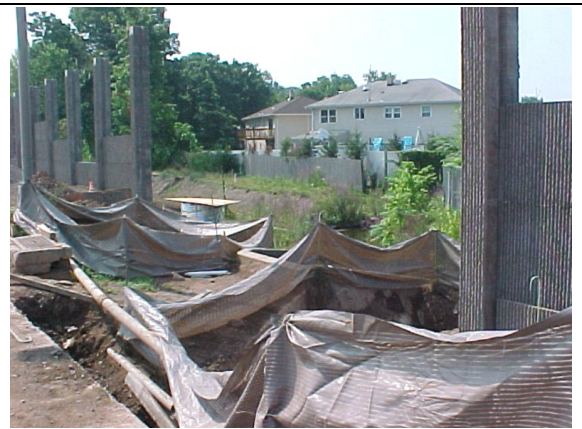
Installation of plastic sheets for soil erosion and sediment control measures.
