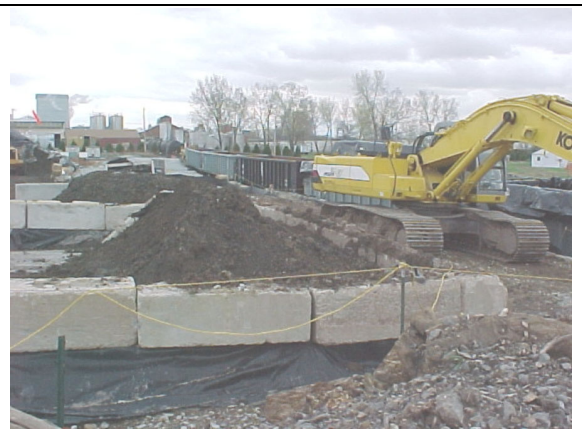
Soil in temporary storage bins awaiting placement into railcars by excavator.
