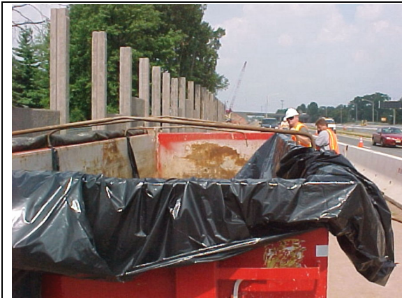
Workers installing liner in roll-off container before loading soil.
