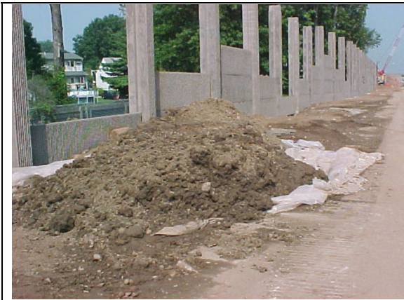
Soil storage pile from excavation for sound barrier installation.
