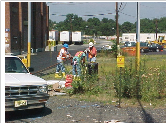
Making preparations for connecting new water line to the existing hydrant.
