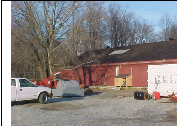
Building 76 on MISS – Location of Soil Sample Preparation Laboratory.
