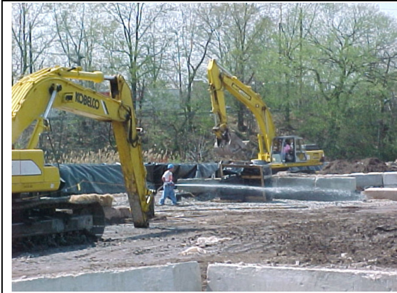
Dust control measures during soil load-out. Excavator loading railcar in distance.
