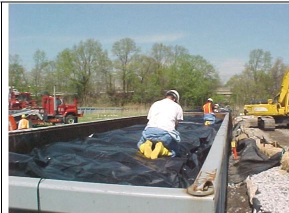
Workers in railcars securing liners before rail shipment.
