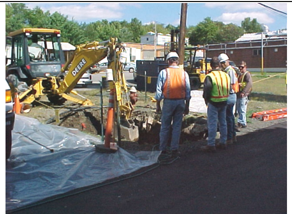
Using excavator to dig trench for water line installation.
