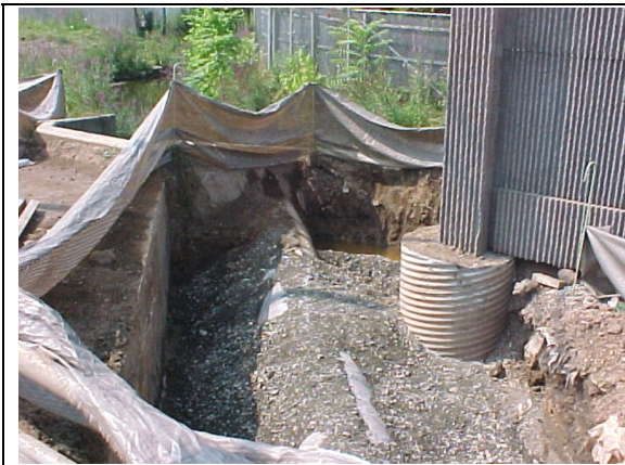
Excavation for installation of caissons to anchor sound barriers.
