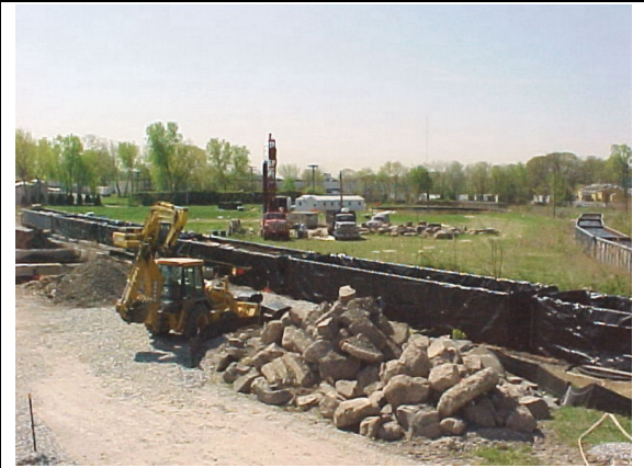
Railcars with liners awaiting loading of soil for off-site disposal.
