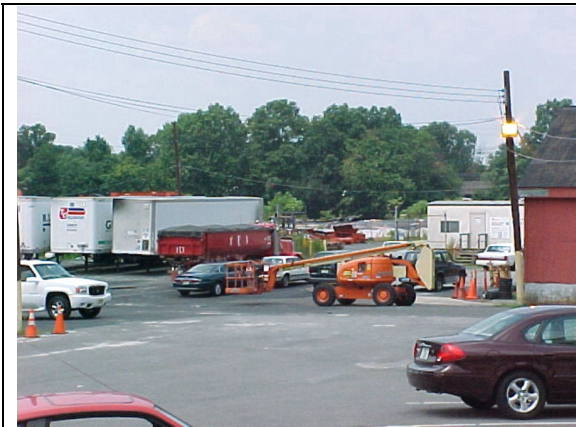
Truck arriving at MISS with contaminated soil from excavations for sound barrier installations along Interstate 80.
