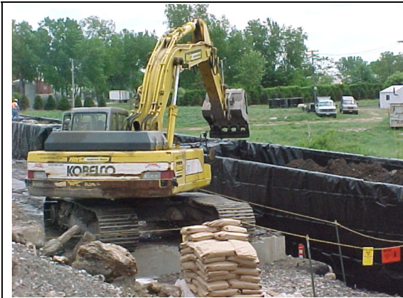
Loading of soil by excavator into railcars containing liners.
