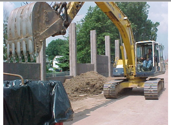
Excavator loading soil into container with liner.
