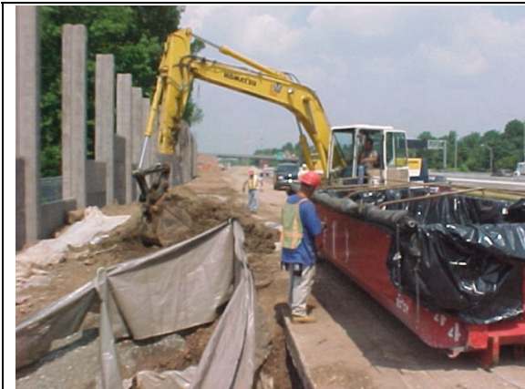
Excavator removing soil from storage pile for placement into container.
