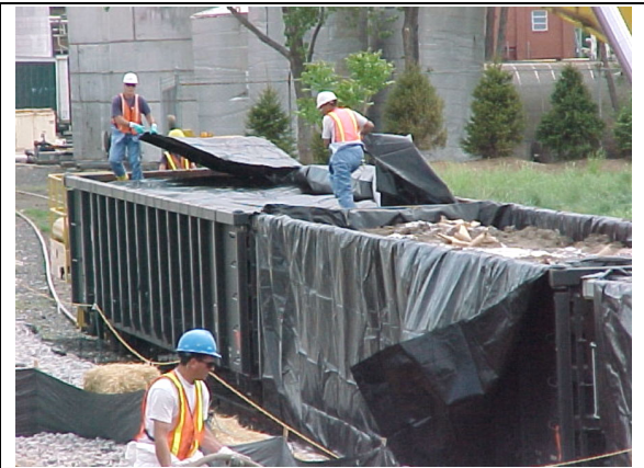
Workers in railcars closing liners before shipment.
