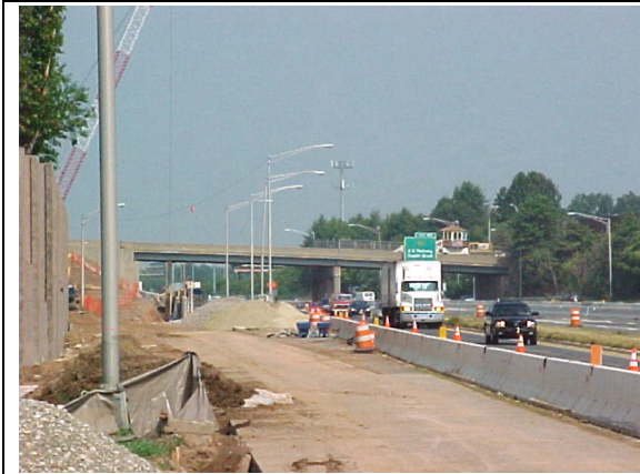
Interstate 80 – Work area for installation of sound barriers.
