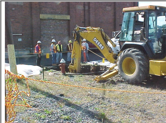
View looking south from trailer office complex of trench excavation.
