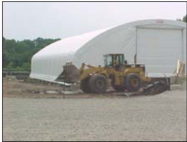
Front-end loader is use to transport soil from inside fabric structure to load-out bins near rail cars.
