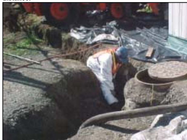
Establishing connection of sewer line to grinder pump manhole at MISS.
