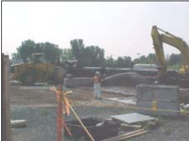
Excavator removing soil from load-out bins and placing into rail cars. Water spray used for dust control.
