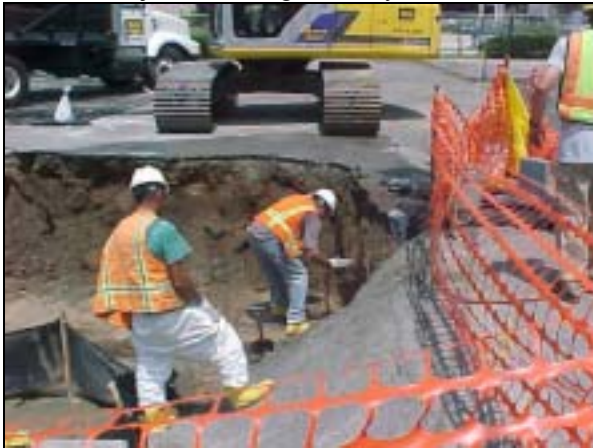
Start of excavation of parking lot at 150 Essex Street.
