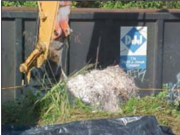
White chalky deposits found in excavated soil for slope cutback similar to material found during lab excavation.
