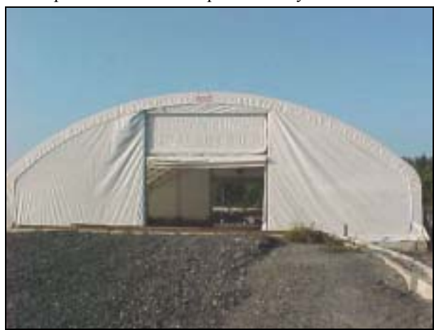
View of empty fabric structure at MISS after completion of successful soil load-out.
