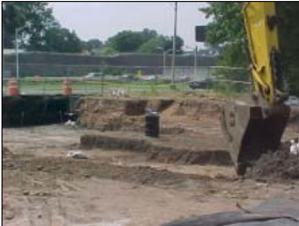
Excavator removing contaminated soil at 160 Essex Street and adjacent I-80 right-of-way.
