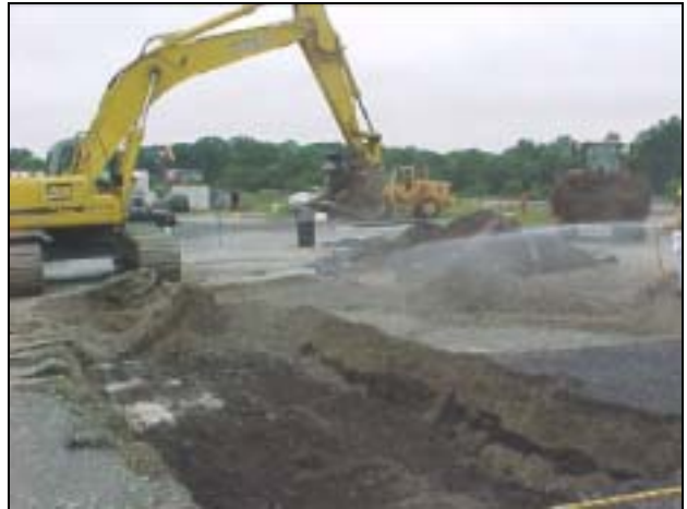
Excavation continues. Water spray was used for dust control.
