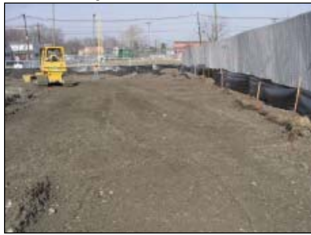
Bulldozer is backfilling the excavated areas at Cluster No. 1.
