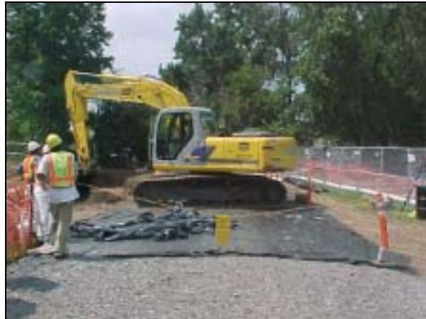
Repositioning loading pad for trucks to continue excavation at 160 Essex Street.
