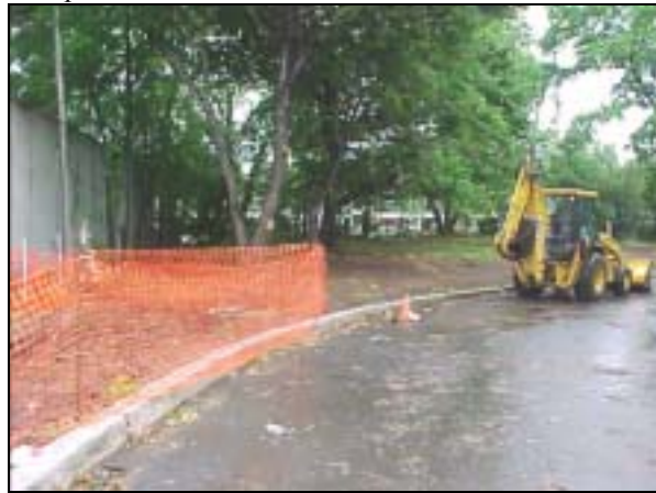
View of I-80 right-of-way after completion of the removal action.
