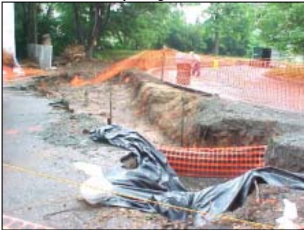
Excavated area along I-80 right-of-way.
