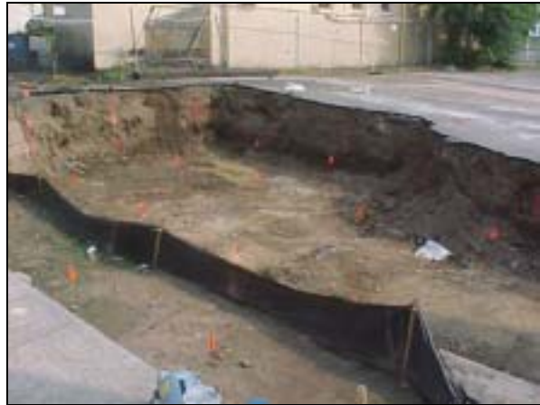
Completed excavation at 150 Essex Street.
