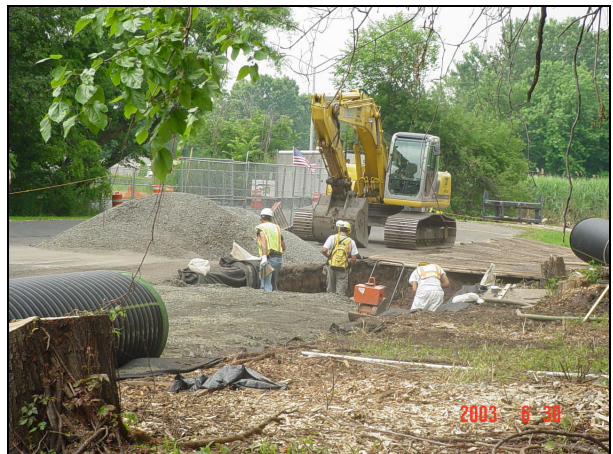
Installation of final sections of HDPE pipe.
