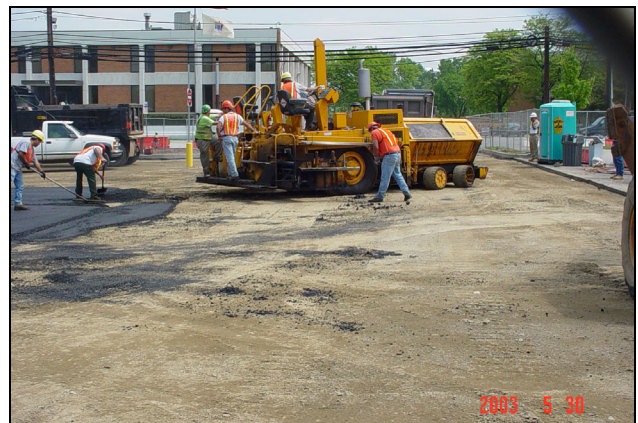
Asphalt repaving in progress at parking areas.
