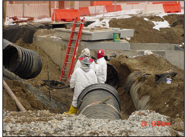
Installation of temporary diversion piping and diversion structure.
