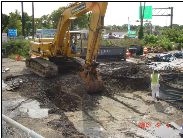
An excavator removing soil from the parking areas.
