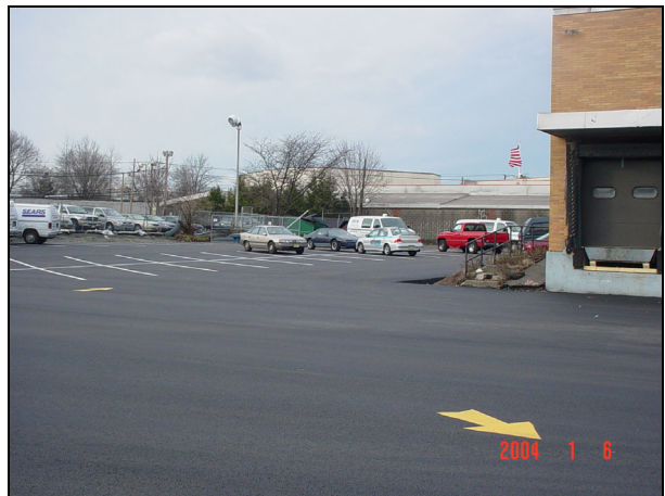
Completion of asphalt repaving and restriping.
