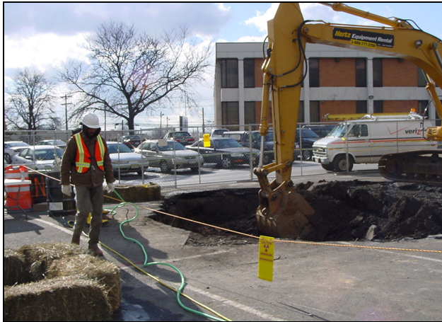
An excavator removing soil from parking area at 113 Essex Street.
