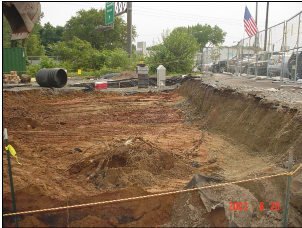
Excavated area at 200 NJ Route 17 South.
