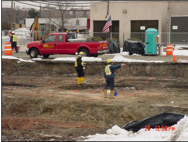
Excavation performed in parking areas at 160-174 Essex street properties.
