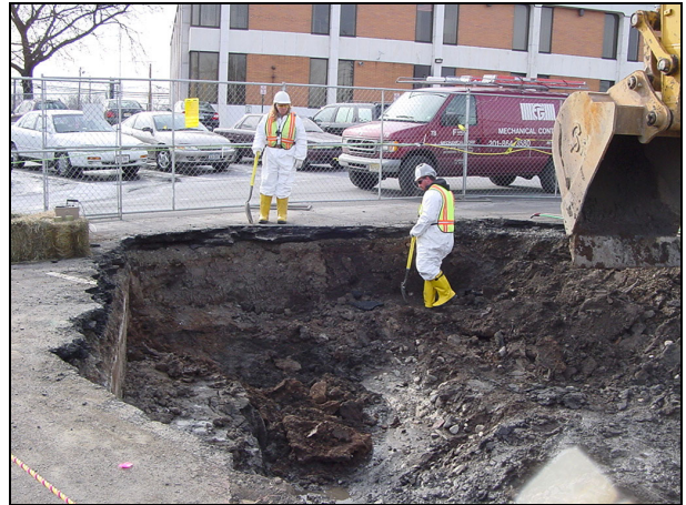
Continuation of excavation from the parking areas.
