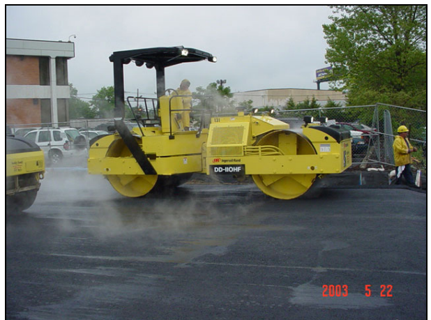
Asphalt repaving in progress in the parking areas at 113 Essex Street.
