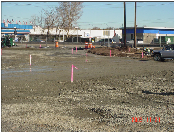
Final grade established in preparation for asphalt repaving.
