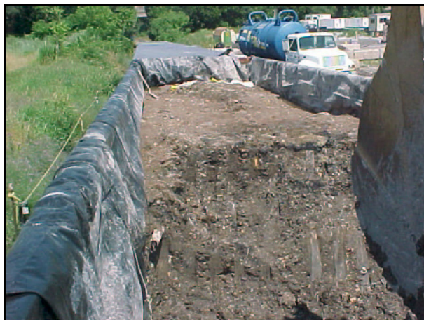
View of partially loaded rail car. When full, the liner will be closed and tied to prevent soil loss during shipping.
