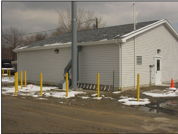
View of west side of radiochemistry laboratory at the MISS. The exhaust stack for the fume hoods is visible.
