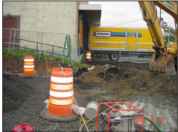
Pumps are used to remove accumulated water in the excavation.
