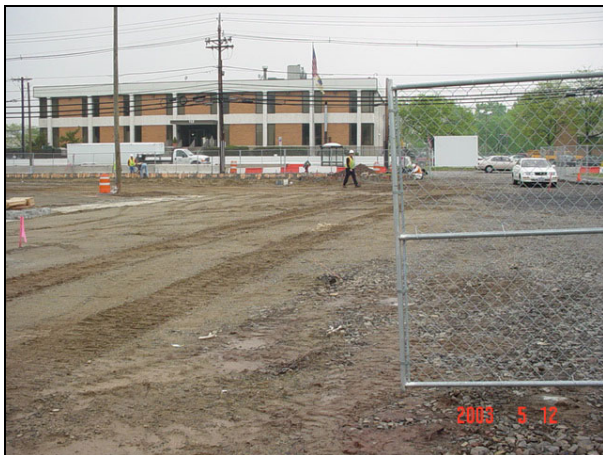
The establishment of final sub-grade for asphalt repaving.
