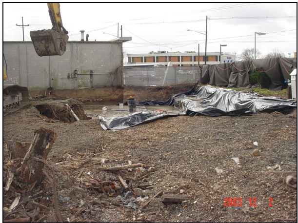
Debris is visible from excavation. A vibrating screen was used at the MISS to remove debris from the soil.
