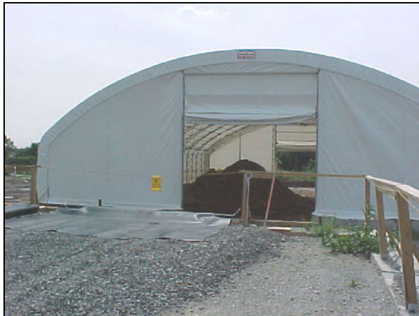
Soil stockpile stored inside fabric structure at MISS prior to start of load-out activities.
