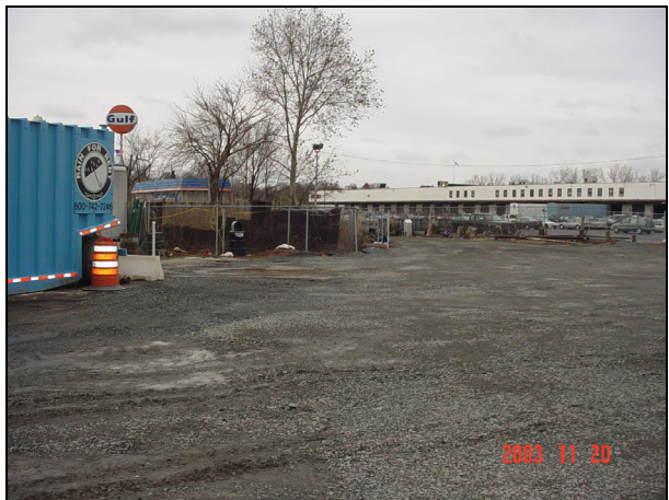
Final grade has been established at the property.
