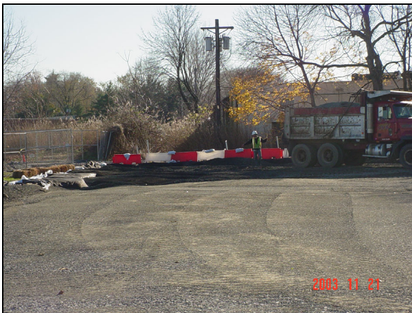
A dump truck is unloading backfill for the excavated areas.
