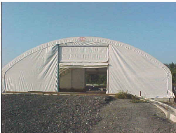
View of empty fabric structure at MISS after completion of successful soil load-out.
