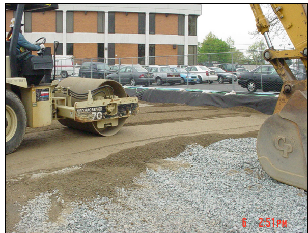
Backfilling and compaction is being performed at the excavated areas.
