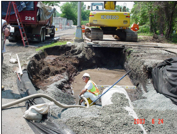
The excavated soil was placed into a lined dump truck for transport to the MISS for disposal.
