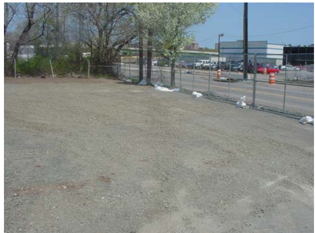
Restoration of the final grade before repaving the lot with asphalt.
