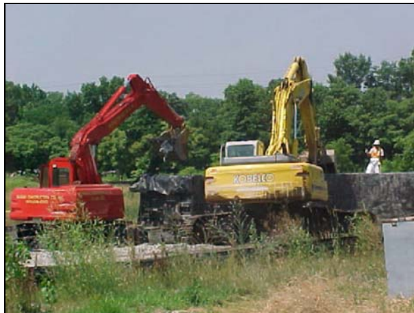
Excavators loading soil into rail cars from storage bins for shipment to off-site disposal facility.
