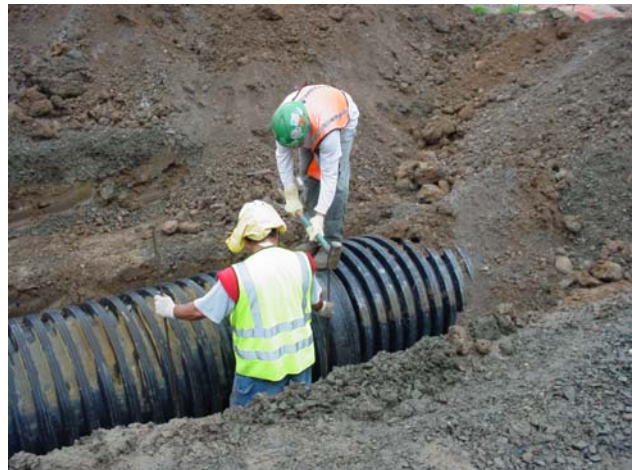
Workers connect the sections for the by-pass line.
