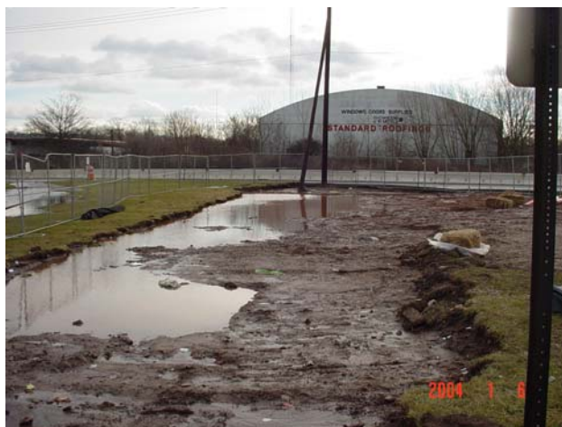
Rain water collected in the excavation while awaiting backfilling.
