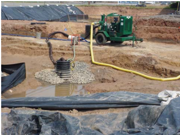
A temporary drain was installed to pump water from the excavation.
