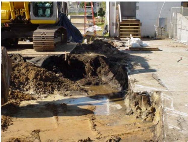
Excavation being performed along the southwest corner of the building.
