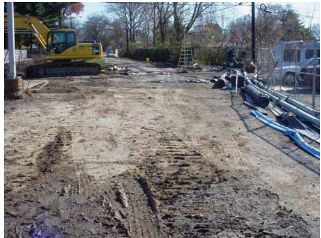
View of the dump truck access road on the site
