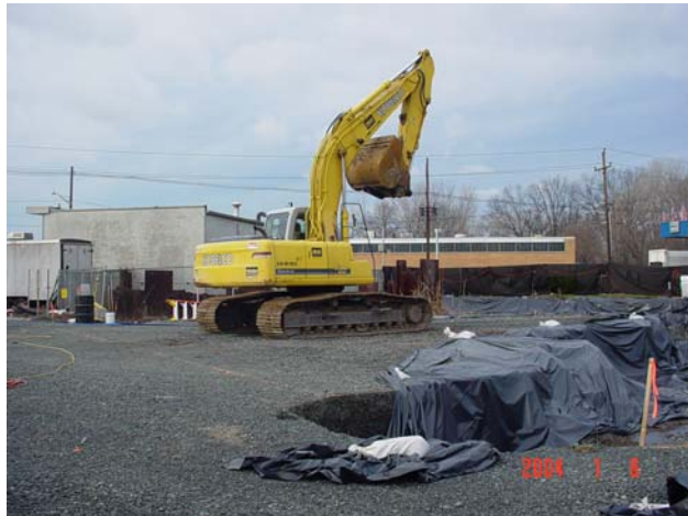
The start of excavation activities at the 167 NJ Route 17 property.
