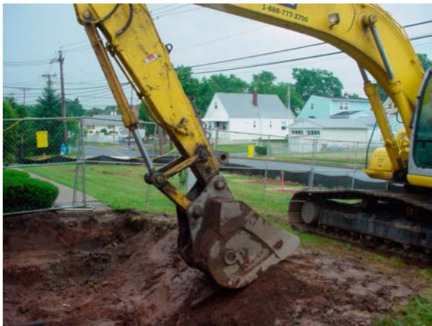
Excavation at the property located at 80 Hancock Street.
