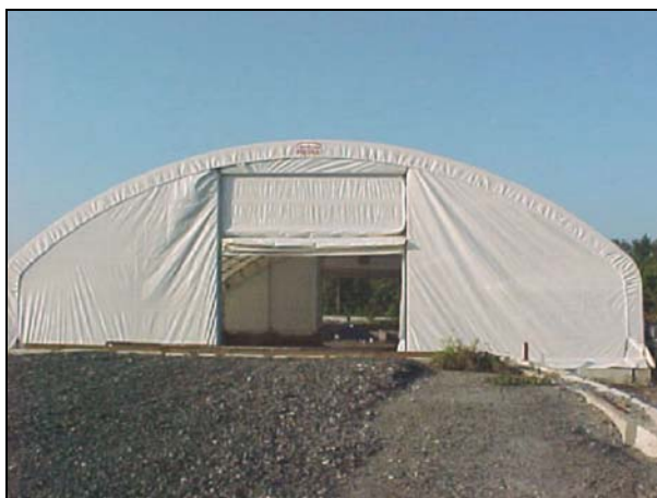
View of empty fabric structure at MISS after completion of successful soil load-out.
