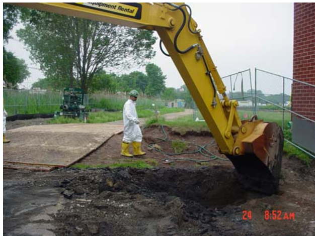
Excavation in progress at the property located at 23 West Howcroft Road.
