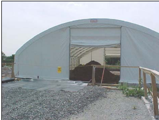
Soil stockpile stored inside fabric structure at MISS prior to start of load-out activities.
