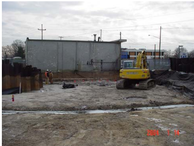
An excavator is used to load soil into lined dump trucks for transport to the MISS for disposal.
