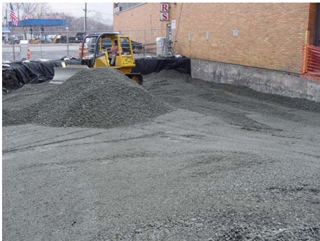
Backfilling being performed on the north side of the building.
