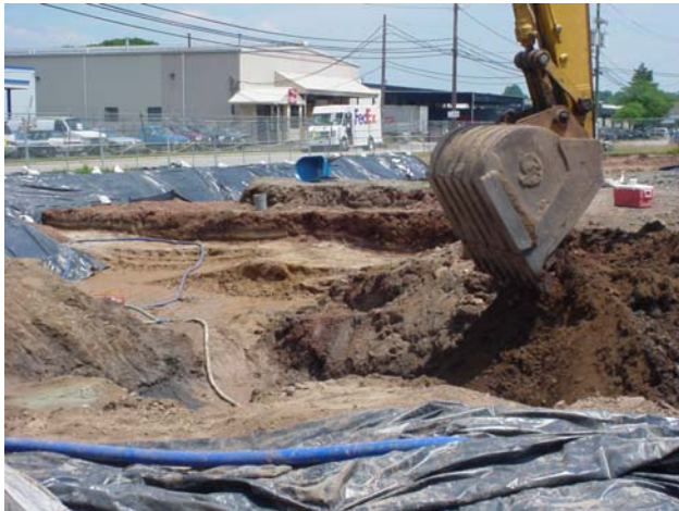
Excavation being conducted at the property located at 80 Industrial Road.
