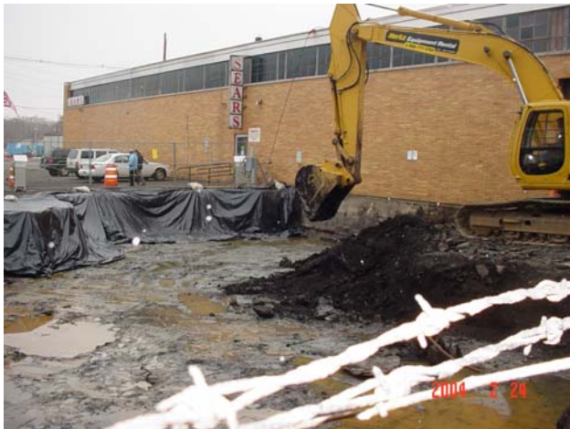
Excavation activities being conducted on the north side of the building.
