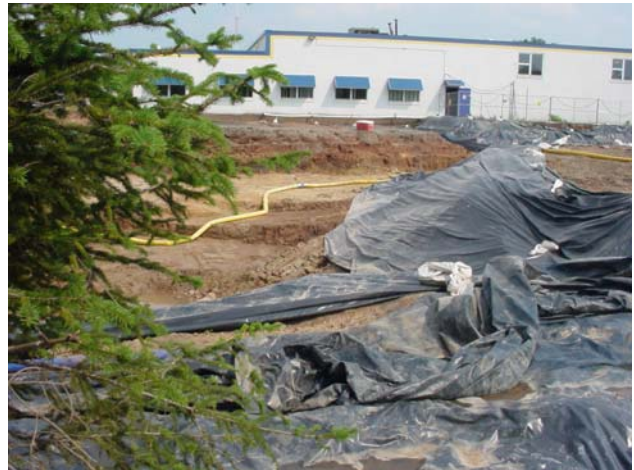
Polyethylene sheets were used to cover the impacted soils.
