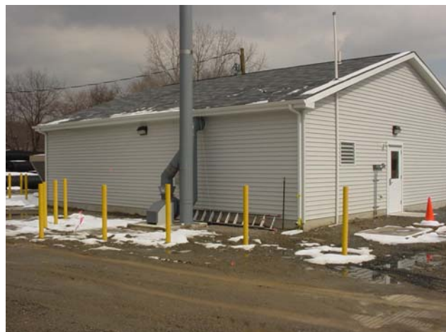
View of west side of radiochemistry laboratory at the MISS. The exhaust stack for the fume hoods is visible.
