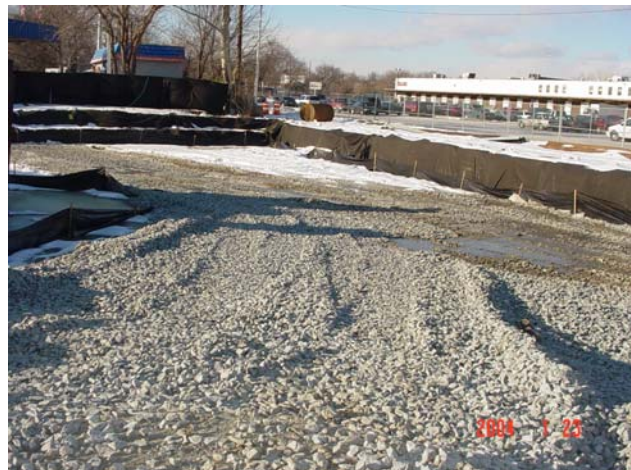
Rough final grade has been established at the property.
