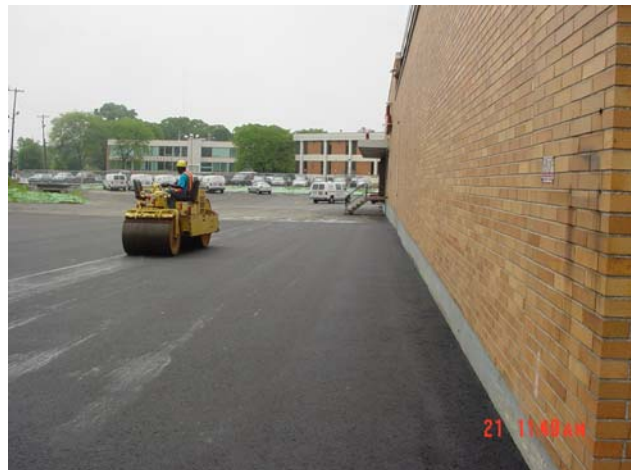
Asphalt paving on the east side of the building.
