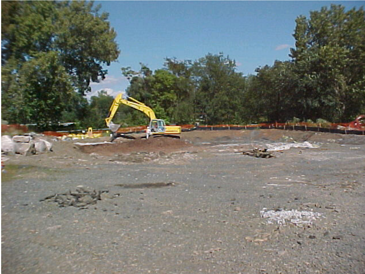
Soil Acquisition Excavation Progress
