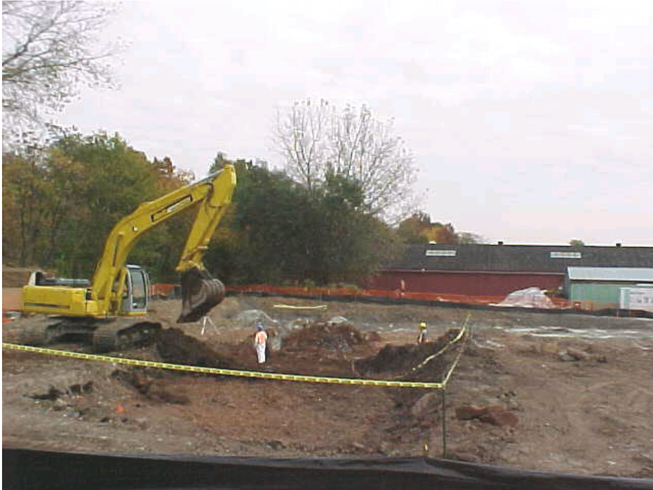
Final Excavation Cut at The Soil Acquisition Area Stage II
