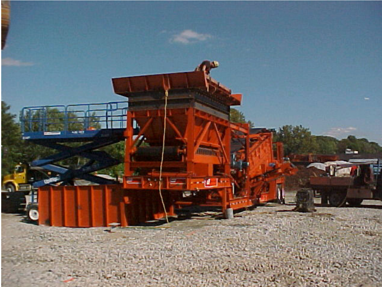
Gravel Separation 2nd Mobilization & Installation
