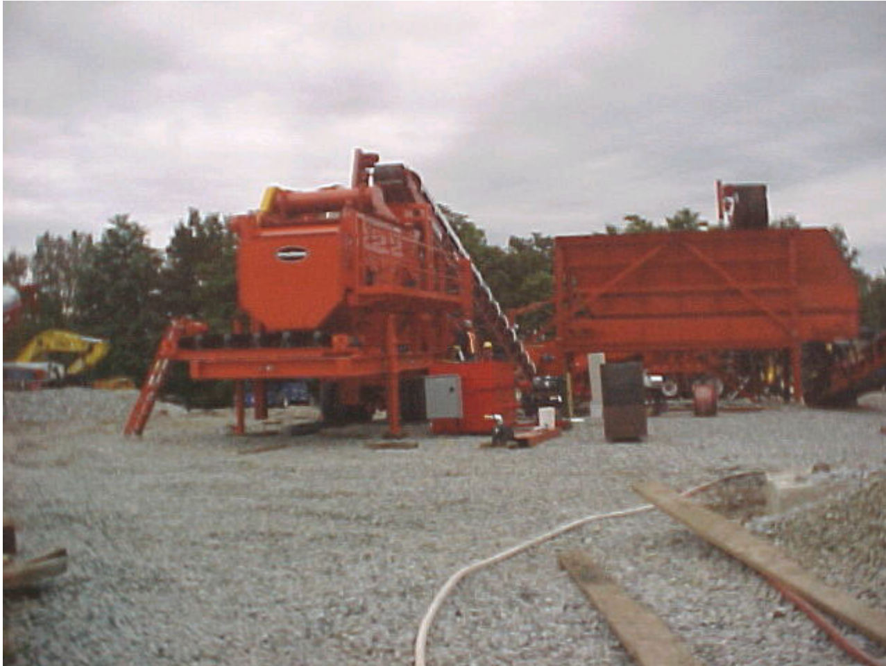
Rinse Unit Installation in Progress
