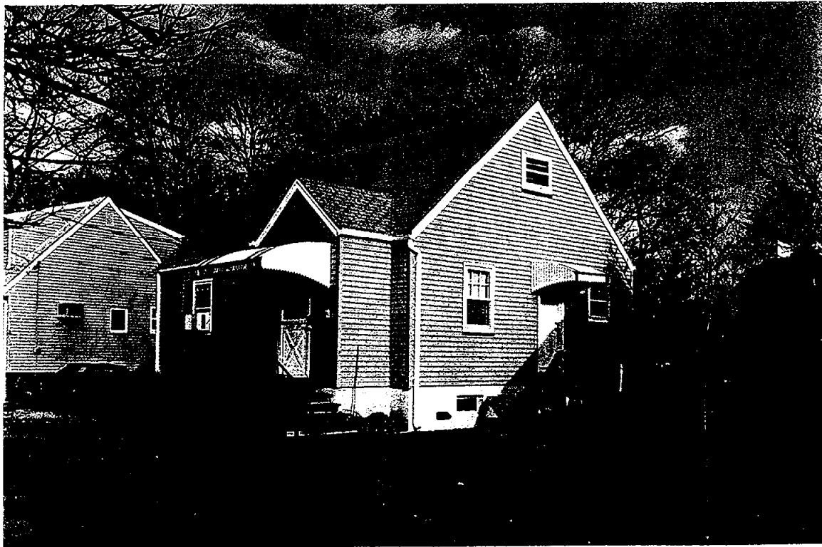
Plate 20. 26 Long Valley Road, Lodi, Facing Northeast
