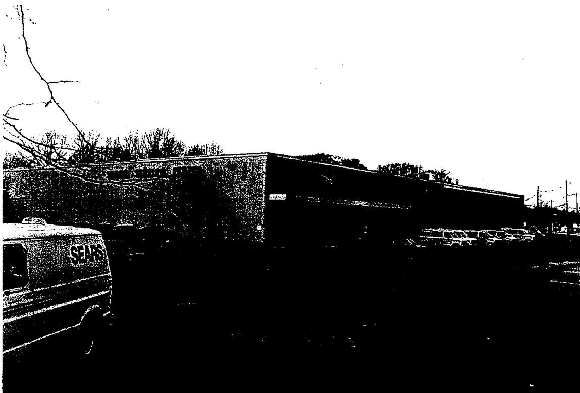
Plate 5. Sears Service Center, 200 Route 17, Maywood, Facing Northwest
