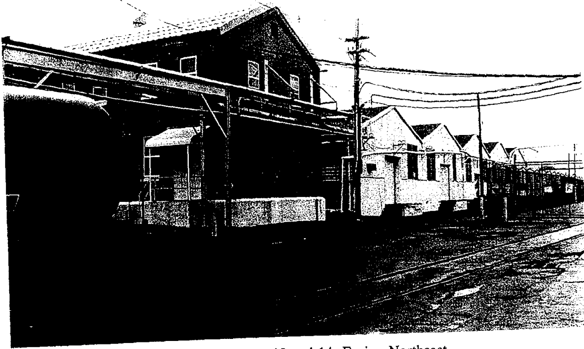
Plate 7. Buildings 13 and 14, Facing Northeast
