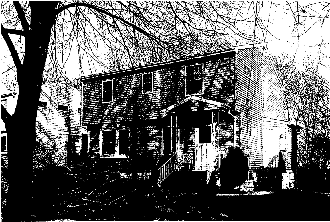
Plate 17. 20 Long Valley Road, Lodi, Facing Northeast
