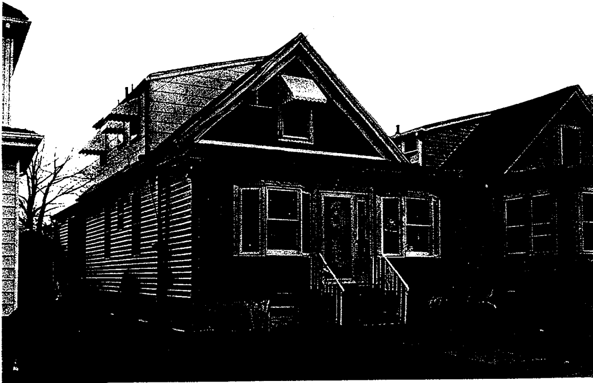
Plate 26. 90 Avenue C, Lodi, Facing Southeast
