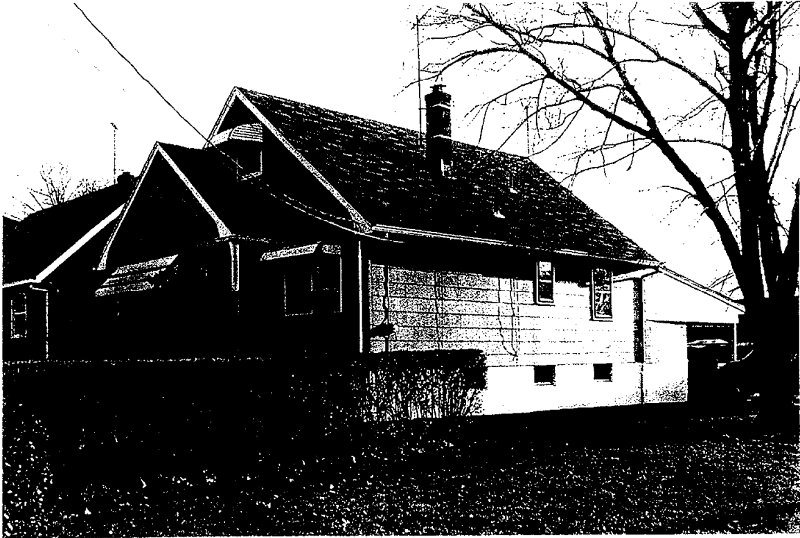
Plate 1. 60 Trudy Drive, Facing Southeast
