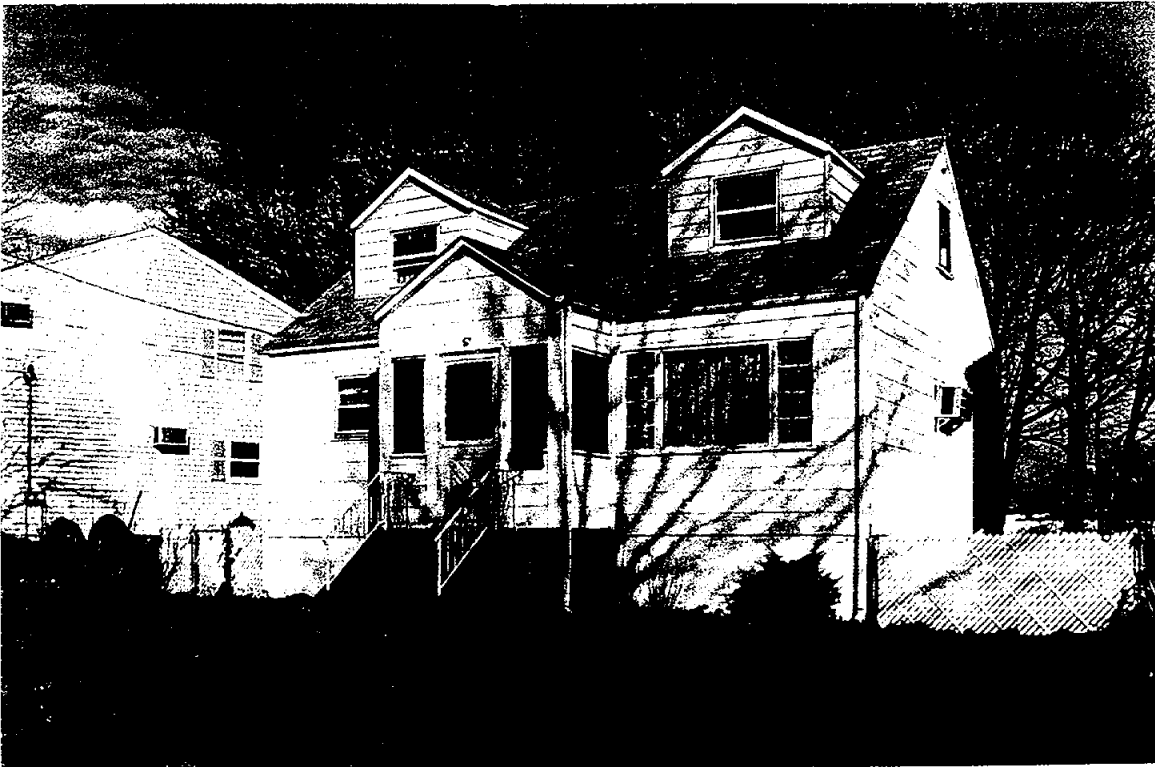
Plate 14. 14 Long Valley Road, Lodi, Facing Northeast
