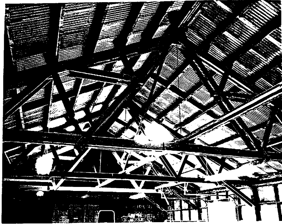
11. Building 76, Ceiling Detail (250°) Not Perspective Correct
