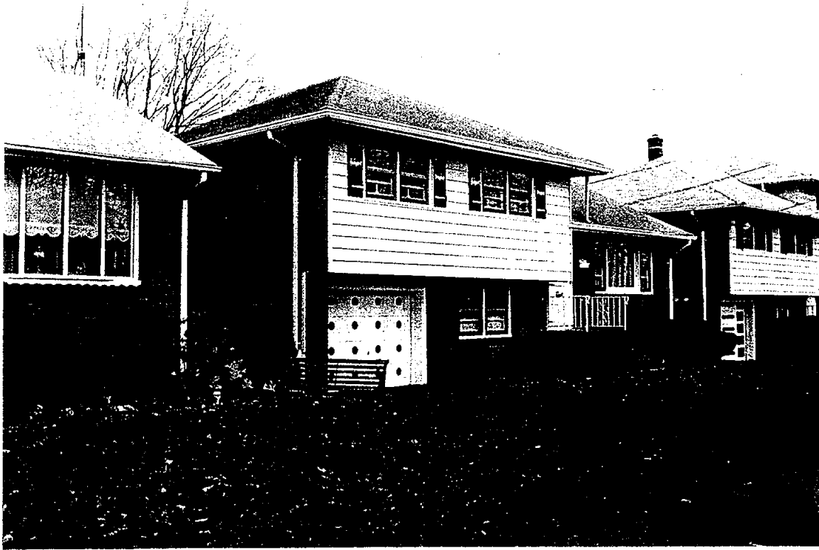
Plate 25. 79 Avenue B, Lodi, Facing Northeast
