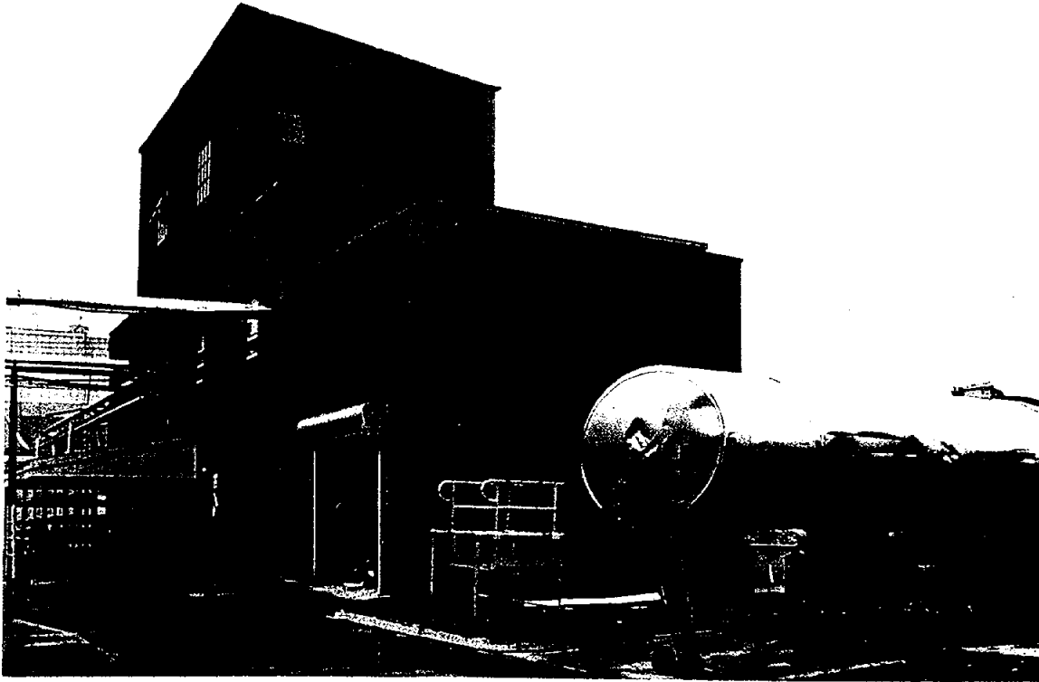
Plate 5. Building 10H, Facing East
