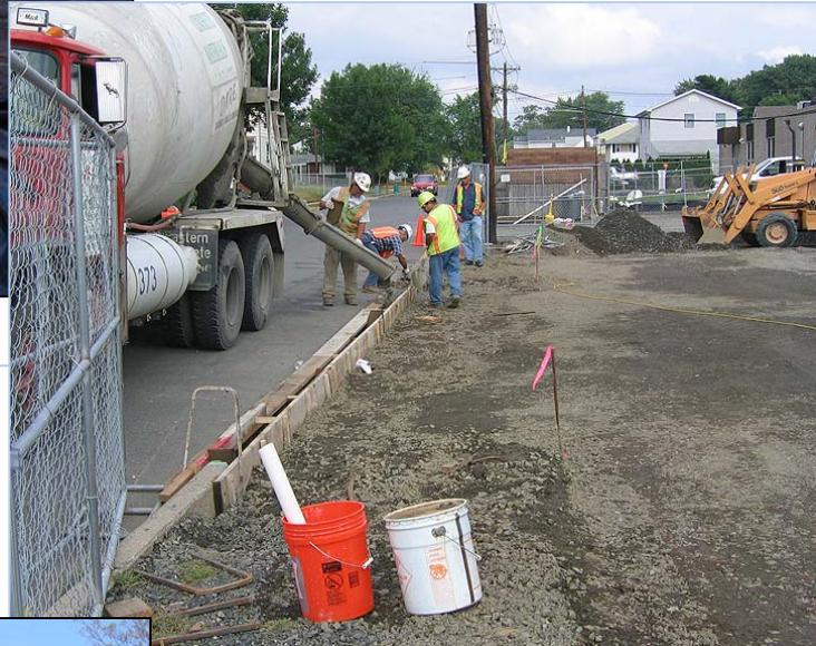
*Excavations are done in discrete areas called survey units, allowing technicians to systematically confirm that cleanup goals have been met prior to backfilling.*
