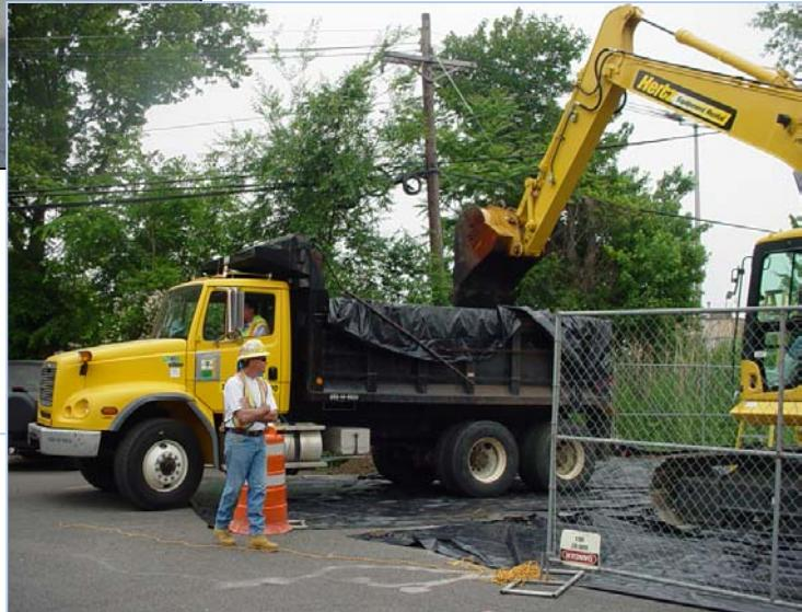
*A truck being loaded with soil at an excavation site. All trucks are checked for residual contamination before leaving work areas.*
