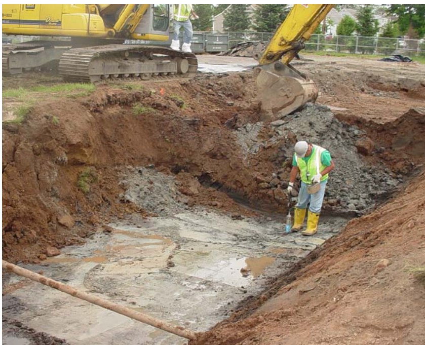
A radiation safety technician taking measurements at a commercial property excavation site.
