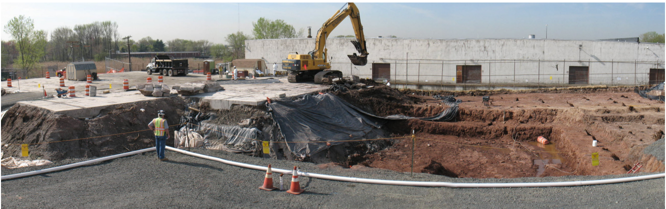
An April 2010 view of soil remediation at one of three waste disposal pits on the 100 West Hunter Avenue, Maywood property. Excavations in this area went as deep as 15 feet.
