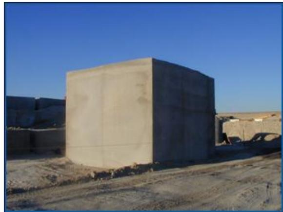
**Figure 3-1. Macroencapsulation of Hazardous Debris**
